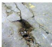
CRACKING & DETERIORATION OF SLAB TOP SURFACE
