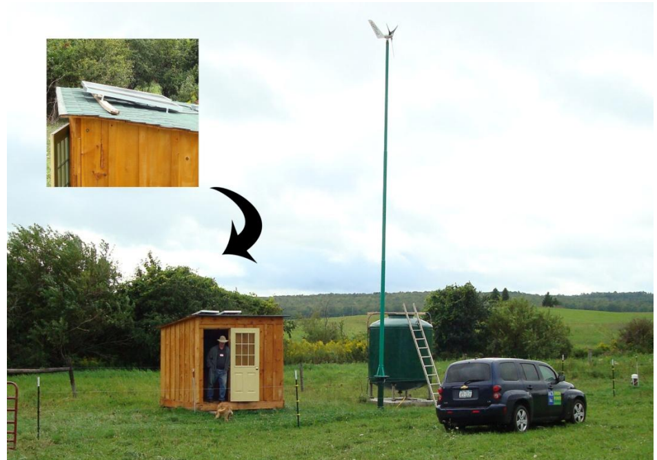
After site testing, a wind turbine and solar panel combination offered the most reliable approach to keeping Jonathan's trough filled with water.
