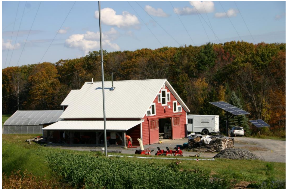
To keep costs down, the Luhrmans installed the wind turbine and solar panels themselves.
